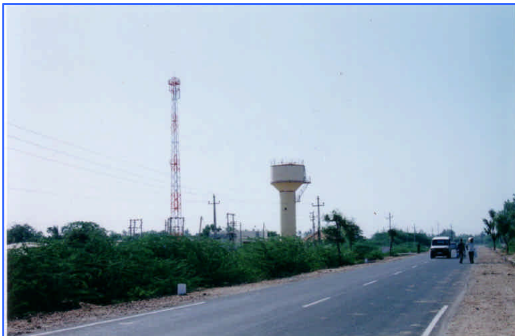
Figure No.26 Gandhidham – Mandvi Highway NH-8A
