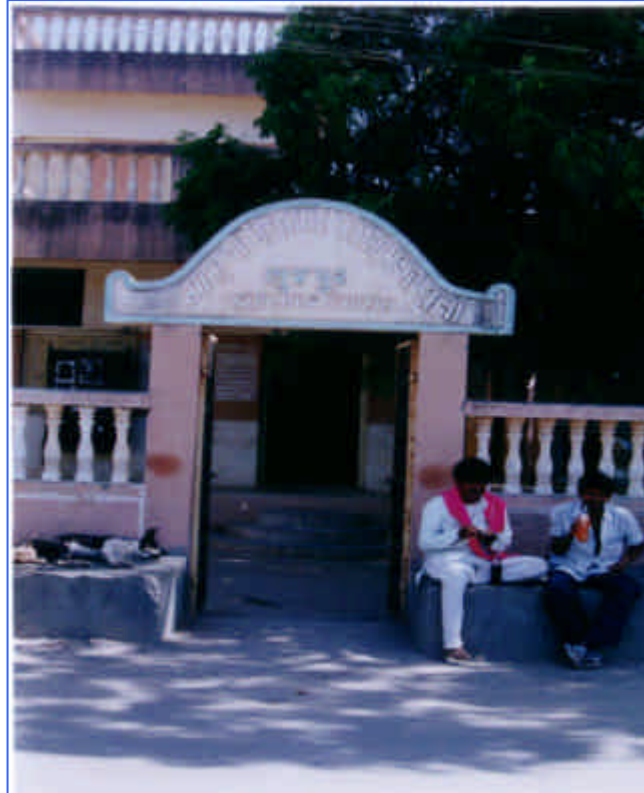
Figure No.3 Gram Panchayat Office, Bhojpar
