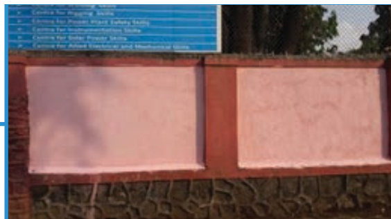
After Application of Paint
