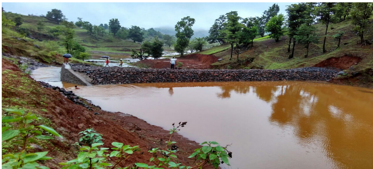
Earthen dam constructed under integrated watershed management intervention, Kadachimate
