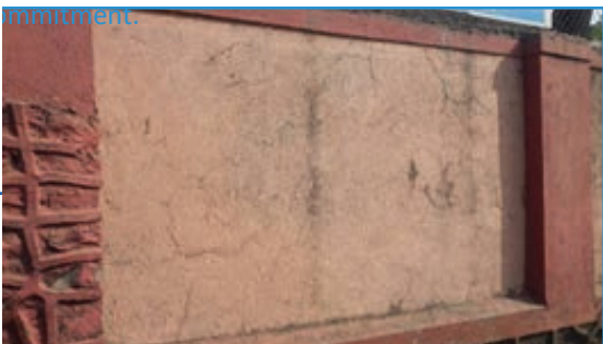
Before application of Paint
