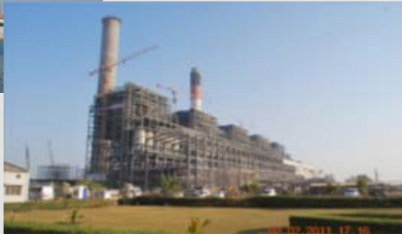
Plant view from Site Office
