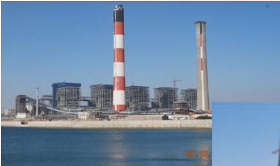
Plant view from Skimmer Bay
