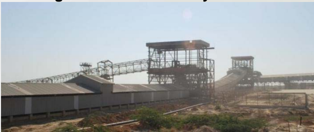
Sheeting work on coal conveyor
