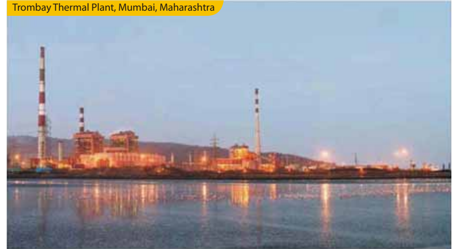
Trombay Thermal Plant, Mumbai, Maharashtra
