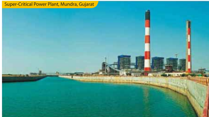
Super-Critical Power Plant, Mundra, Gujarat
