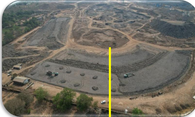
Geomembrane Faced Rockfill Dam
