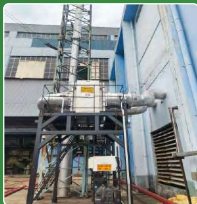
Installation of RECD and De-NOx System at DG set #1 and 2 to reduce the particulate matter, So2 emission and NOx emission
