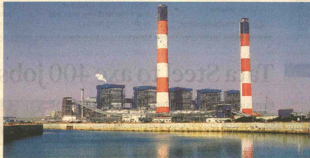
Powering ahead Tata Power's 4,000 MW Mundra Plant
