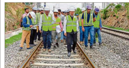
K-RIDE managing director Lakshman Singh and others inspect work on the Kanaka line of the Bengaluru suburban railway project on Sunday.
