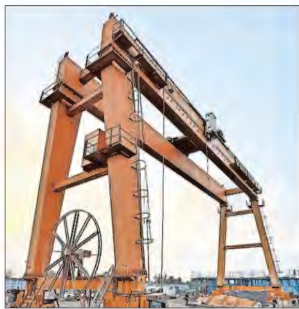
The gantry crane from which the workers fell to their death. EXPRESS
