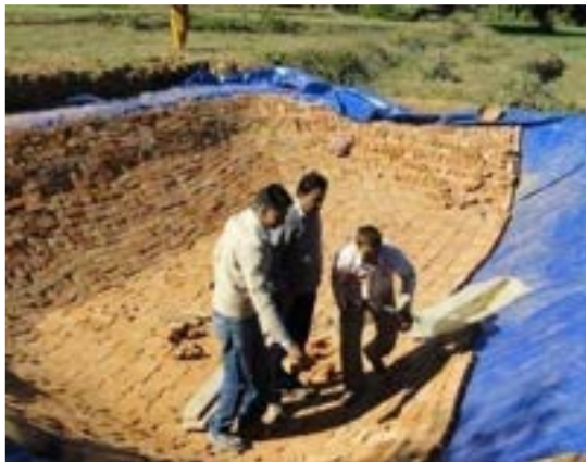
Preparation of polylined tank
