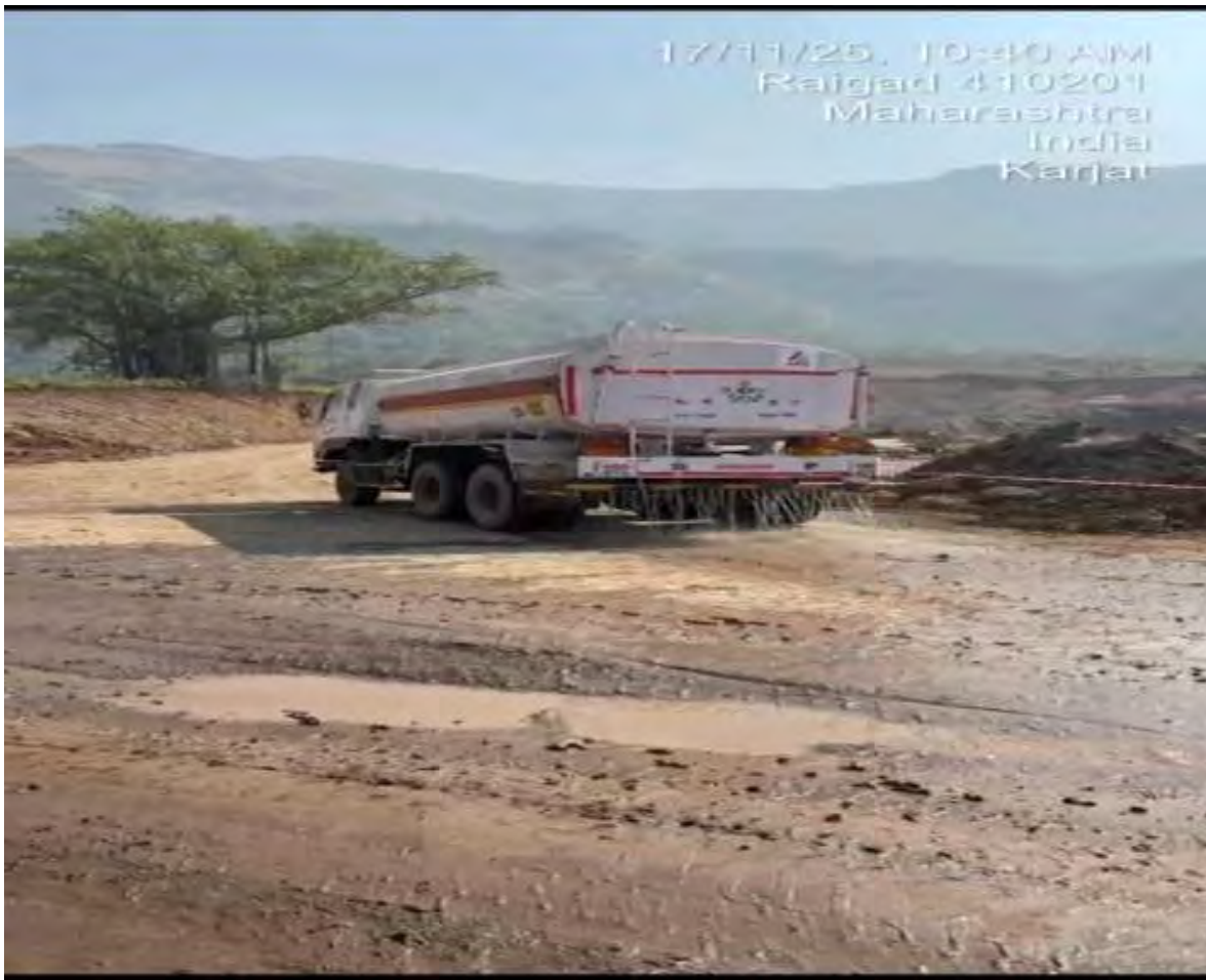
Water Sprinkling On road
