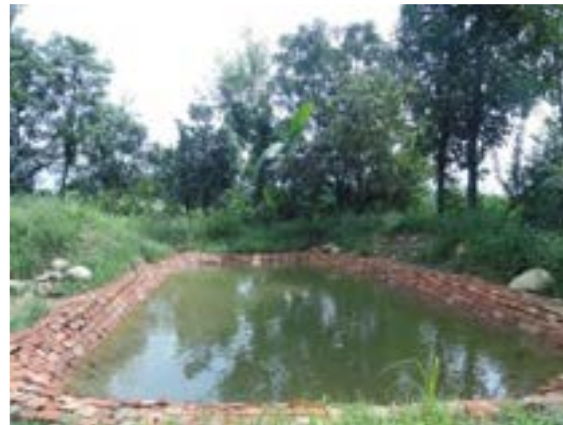
Rain water harvested in polylined tank
