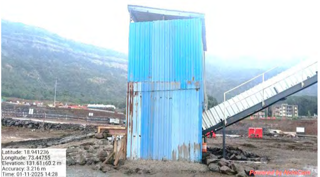
Feeding Hopper Covered
