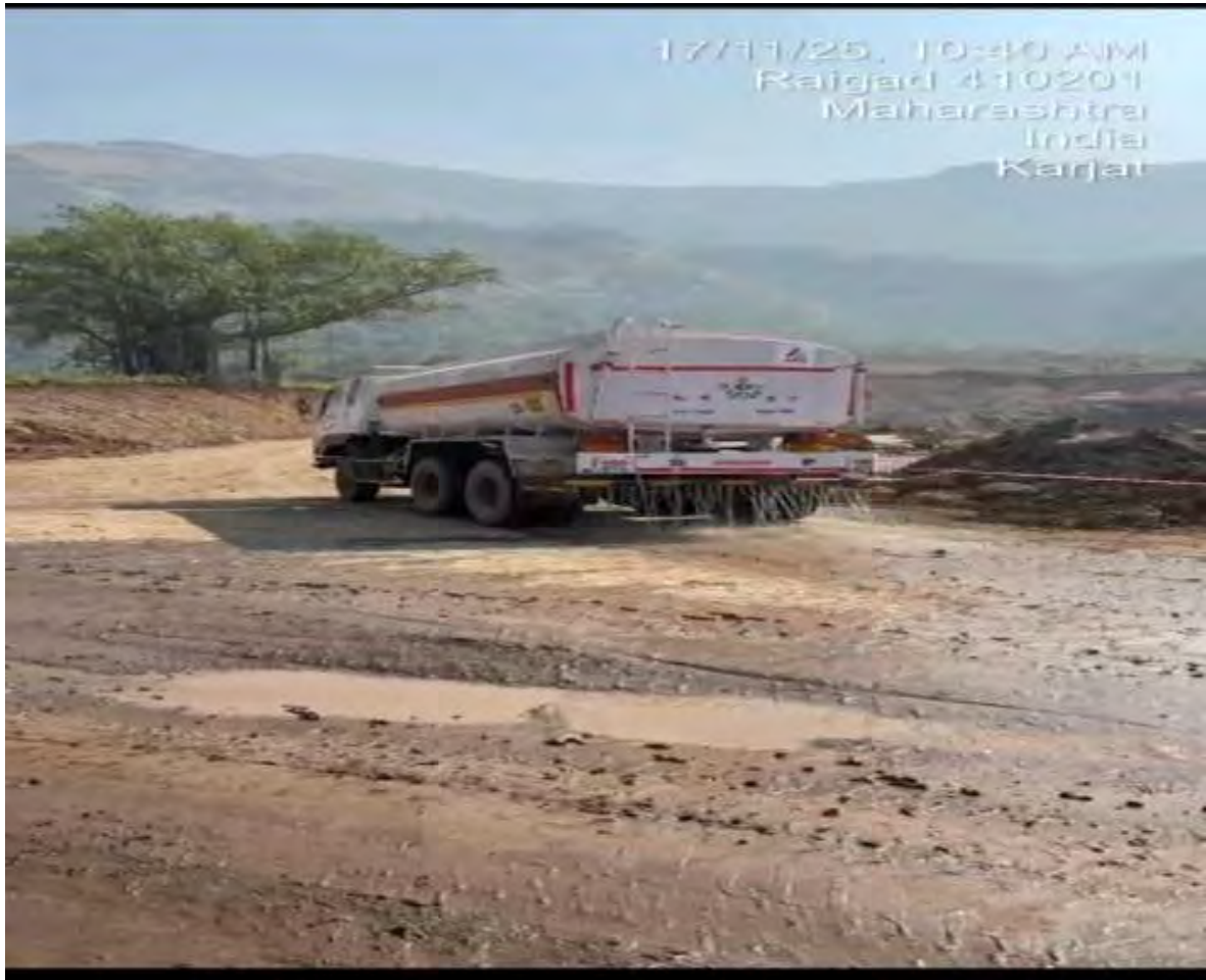
Water Sprinkling On road
